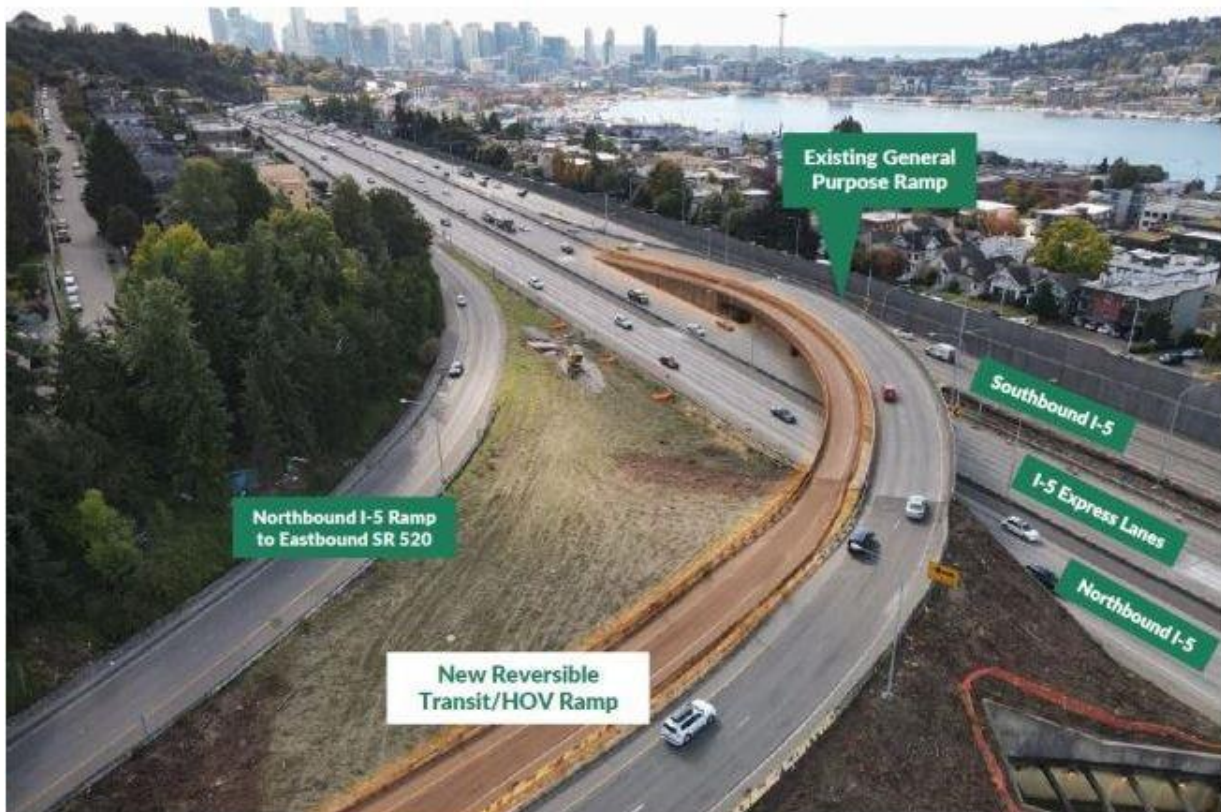
Figure 95: Example of Managed Lane in Seattle
