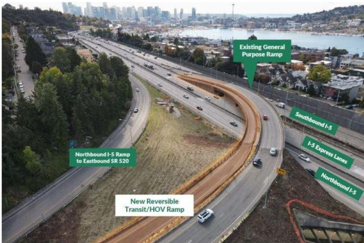
Figure 95: Example of Managed Lane in Seattle
